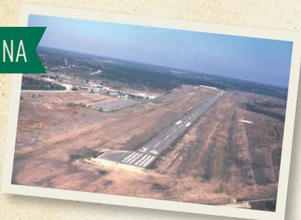
The airport is located one mile north of Ozona. In 1998, a \$2.4 million federal grant was used to upgrade the runway, taxiway, and lighting system. The all-weather hot mix asphalt runway is 6,000 feet in length, 75 feet wide, and will accommodate any aircraft weighing up to 70,000 lbs. There is a very large parking area and radio-controlled lights for strong illumination. G.P.S. IFR Approach OZA (KOZA)
